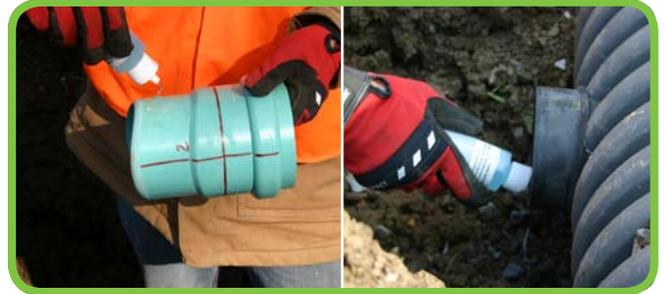
**STEP 5:** Insert the PVC hub into the rubber sleeve. Aligning the red, vertical line on the hub with the gold line on the sleeve. Place a wood block on the hub, and firmly hammer the hub into the sleeve until the sleeve is aligned with the red horizontal line on the hub.
