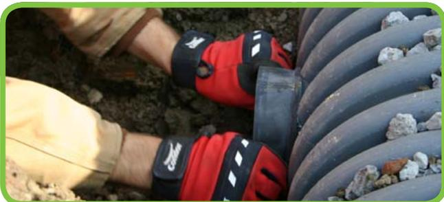
**STEP 4:** Apply the soap solution to the outside of the PVC hub and to the inside of the rubber sleeve.
