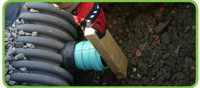
**STEP 6:** Place and tighten the stainless steel band securely over the sleeve.
