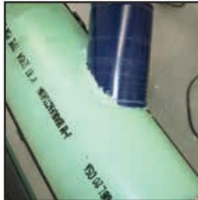
Whether you are cutting a hole for tees or wyes, these guides will keep the pilot bits from "walking", so that you don't ruin the mainline pipe. If you use an Inserta Wye, it is imperative that you cut a teardrop shaped hole.
