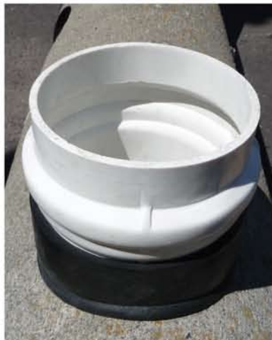
Universal FATBOY® installed into 8" concrete pipe
