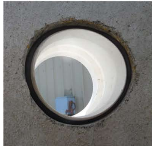
Inside view of Inserta Tee installed in concrete pipe
